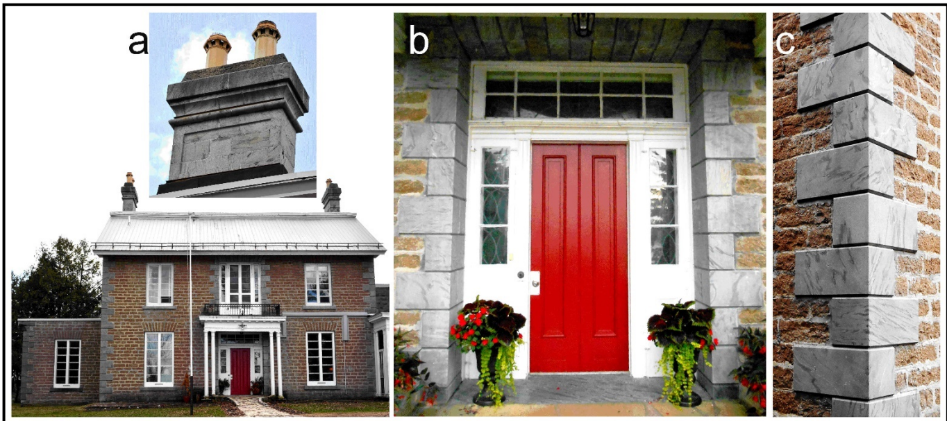
Corners a and b entrance at "The Hill" are framed with Arnprior Marble
