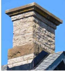
Craig Block chimney
